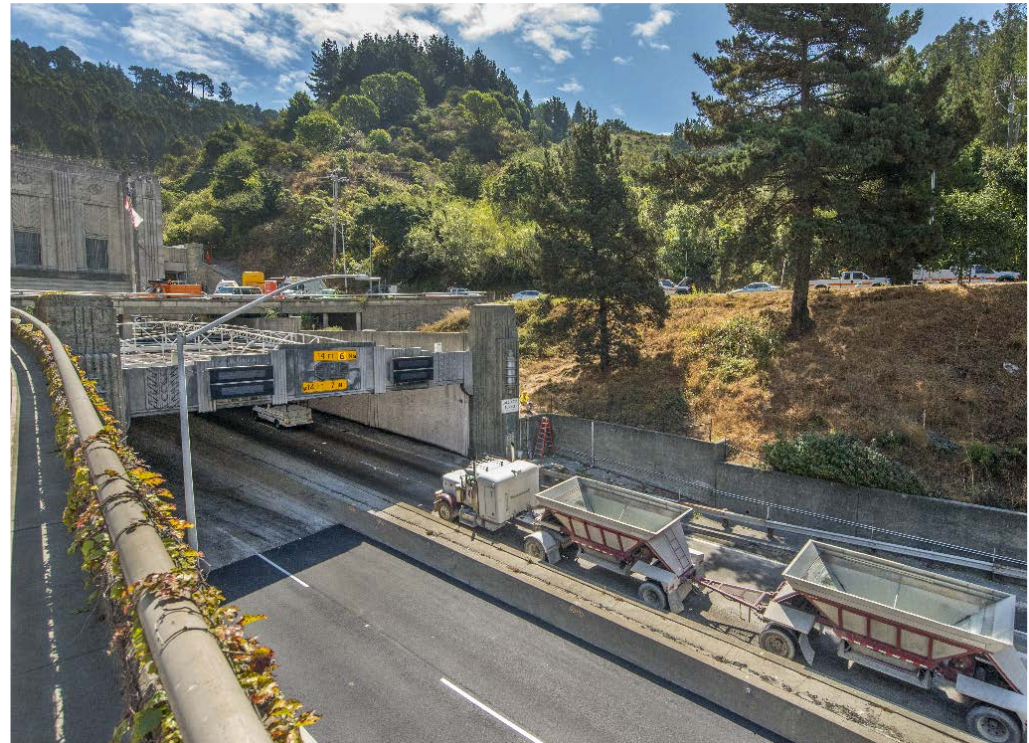
Entering Caldecott Tunnel
